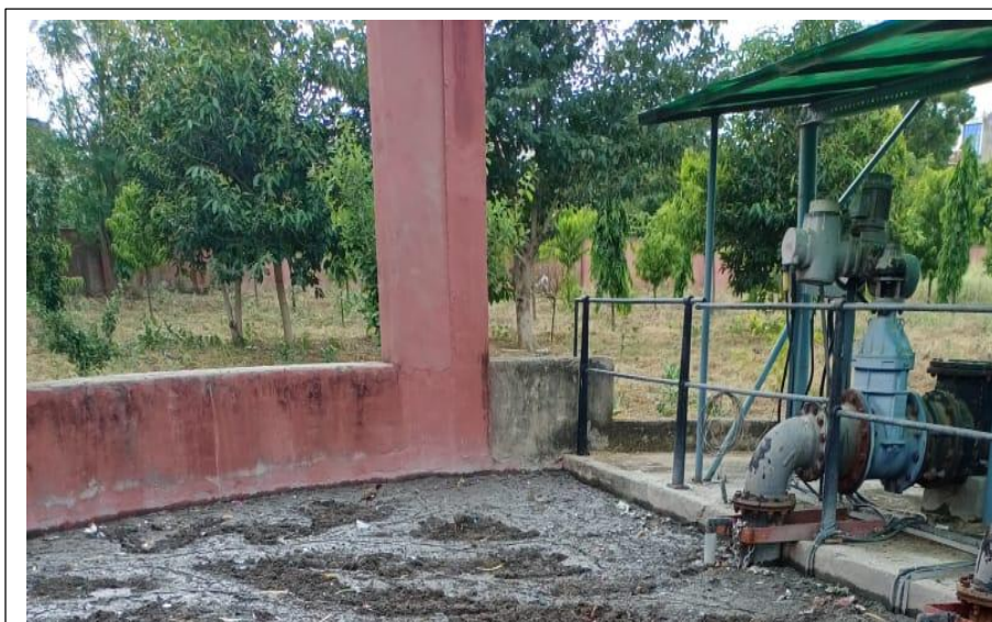
Fig.1 Municipal sludge sample collected from 8 MLD sewage treatment plant, Brahmapuri, Jaipur
